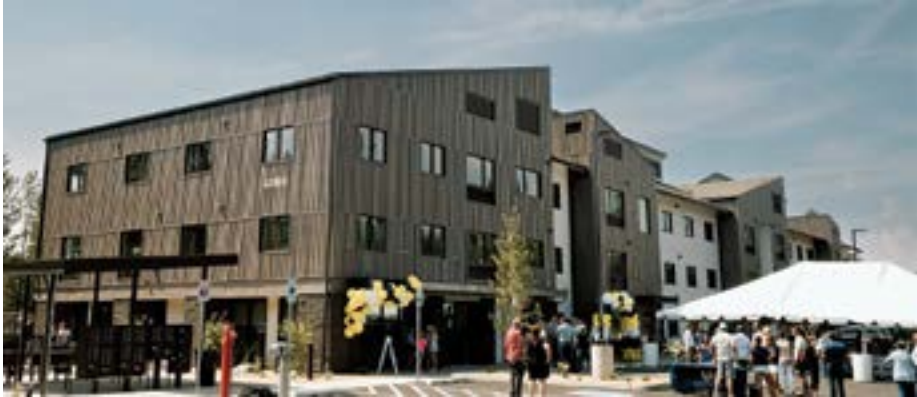
PHASE 1 OF WICKIUP STATION, SHOWN HERE AT THE GRAND OPENING, CONSISTS OF 39 UNITS, WITH TEN RESERVED FOR VETERANS | PHOTOS COURTESY OF FOUNDATION FOR AFFORDABLE HOUSING
