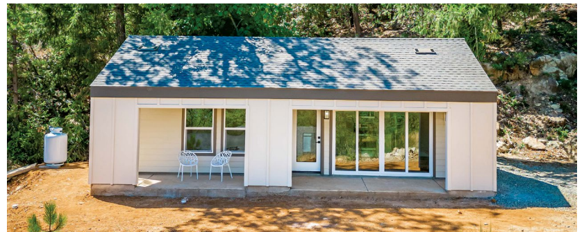
EXAMPLES OF CUSTOM ADDITIONAL DWELLING UNITS BUILT BY ADU SPECIALISTS ANCHORED TINY HOMES, WHICH RECENTLY OPENED IN BEND | PHOTO COURTESY OF ANCHORED TINY HOMES
