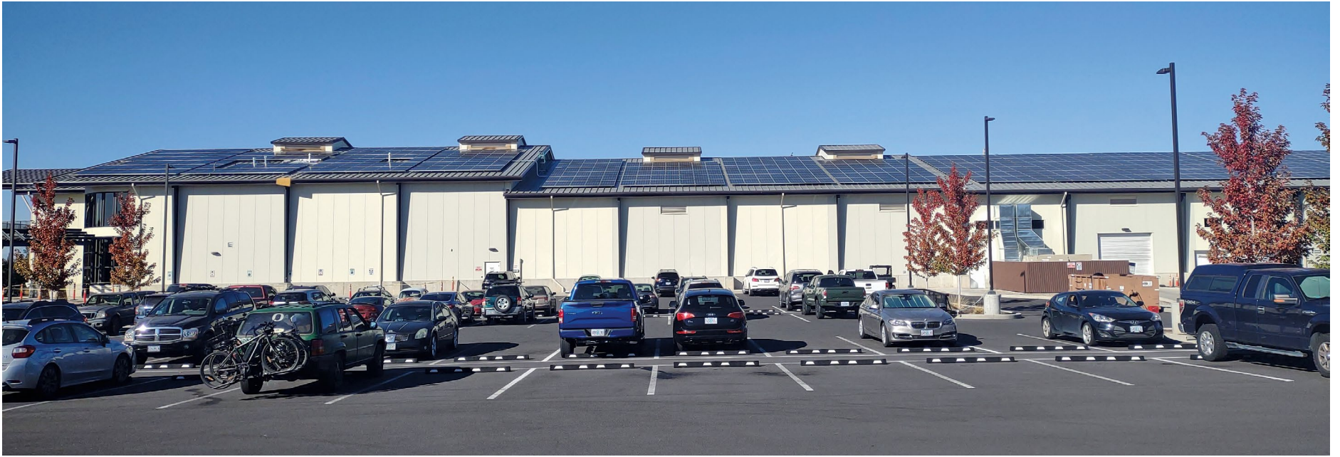
PHOTO | COURTESY SUNLIGHT SOLAR
