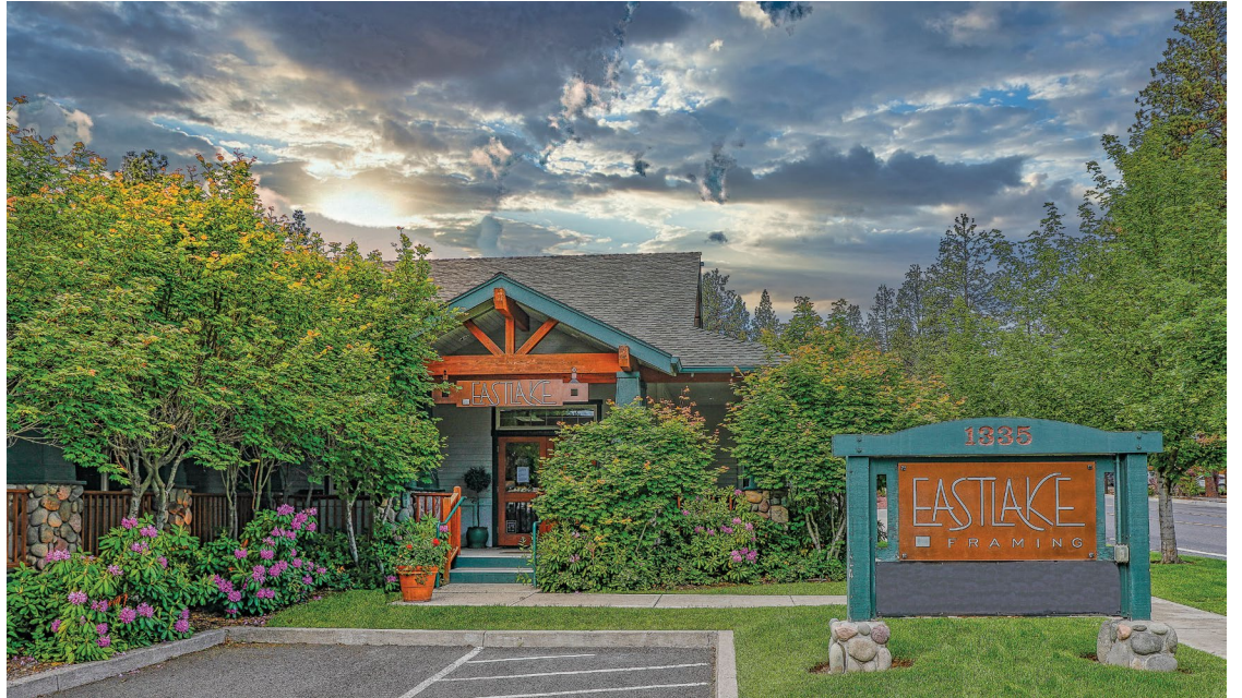
PHOTOS | COURTESY OF EASTLAKE FRAMING
