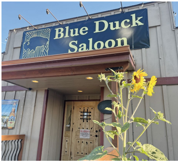
IN ADDITION TO BUILDING A KITCHEN AND RENOVATING THE INTERIOR, BLUE DUCK'S OWNER CONTINUES TO MAKE IMPROVEMENTS
