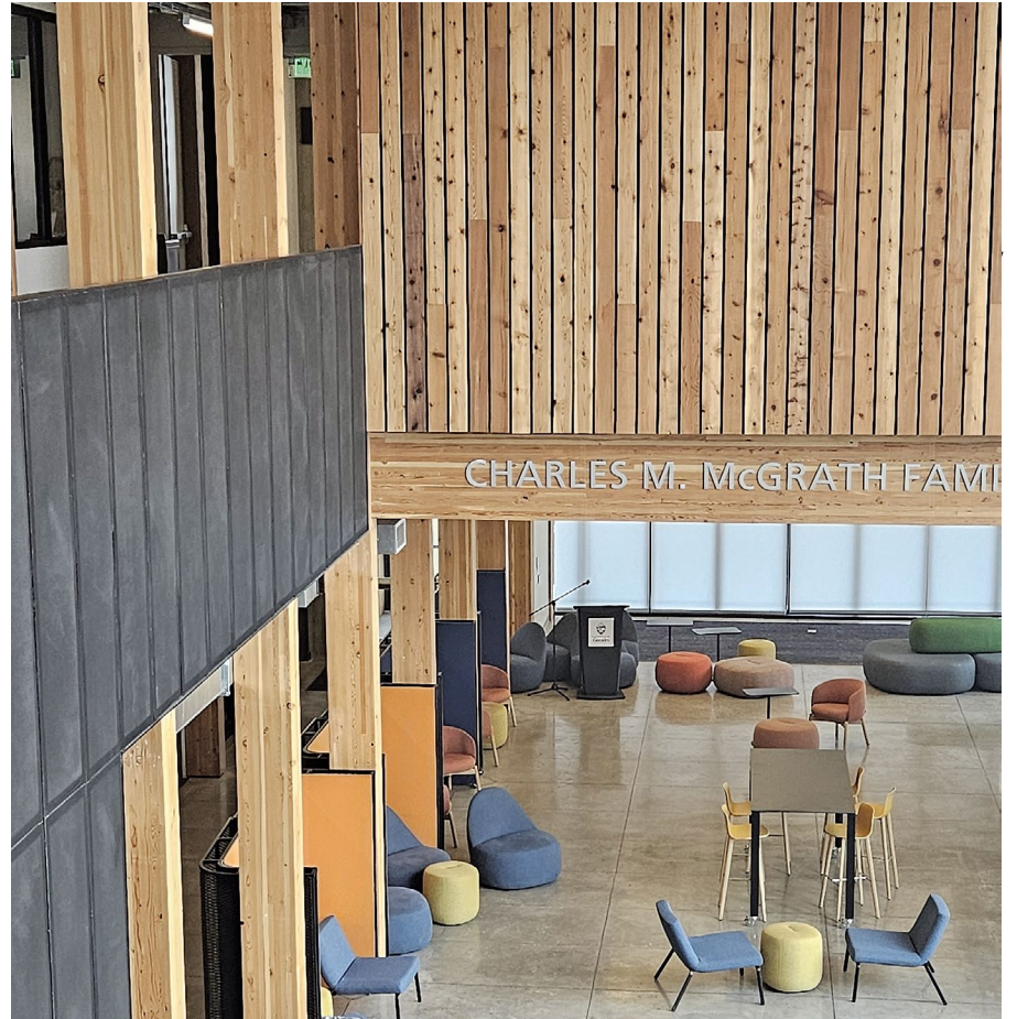
THE USE OF MASS TIMBER, SHOWN HERE IN THE EDWARD J. RAY HALL BUILDING, REFLECTS THE UNIVERSITY’S COMMITMENT TO ENVIRONMENTAL SUSTAINABILITY | PHOTO BY ANDREA HINE
