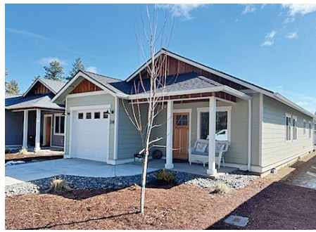
CONSTRUCTION IS UNDERWAY ON FOUR HOMES IN THE WOODLANDS, WITH A TOTAL OF TEN SLATED FOR THIS HABITAT FOR HUMANITY SUBDIVISION
