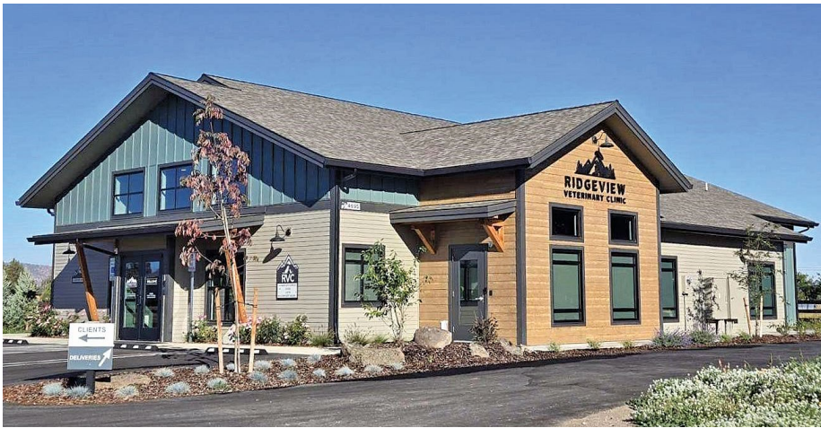
PHOTO | COURTESY OF STEELE ASSOCIATES ARCHITECTS
