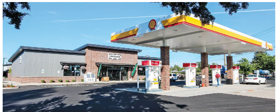
PHOTO | COURTESY OF STEELE ASSOCIATES ARCHITECTS
