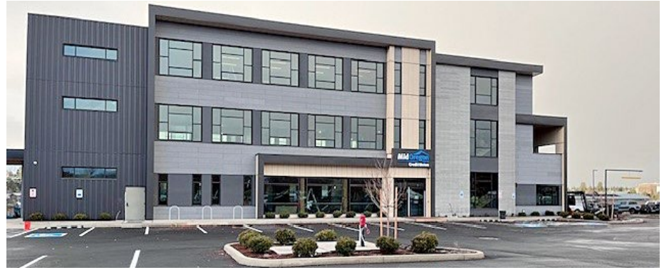
PHOTO | COURTESY OF SUNWEST BUILDERS
