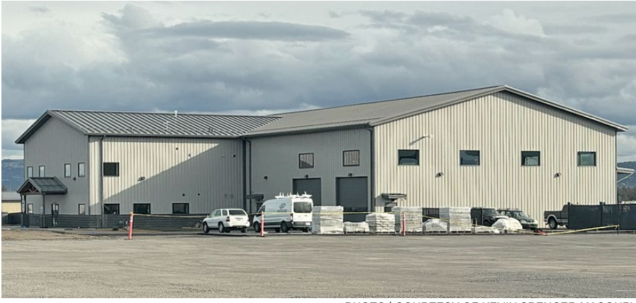
PHOTO | COURTESY OF KEVIN SPENCER MASONRY
