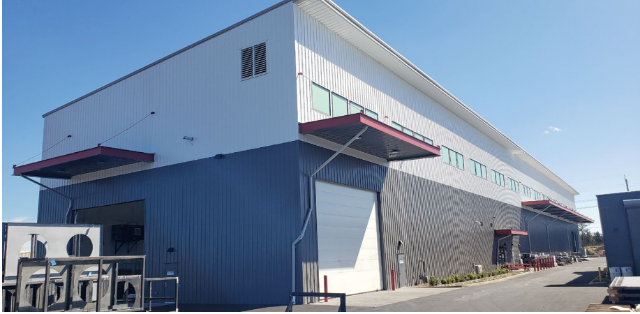
PHOTO | COURTESY OF SUNWEST BUILDERS
