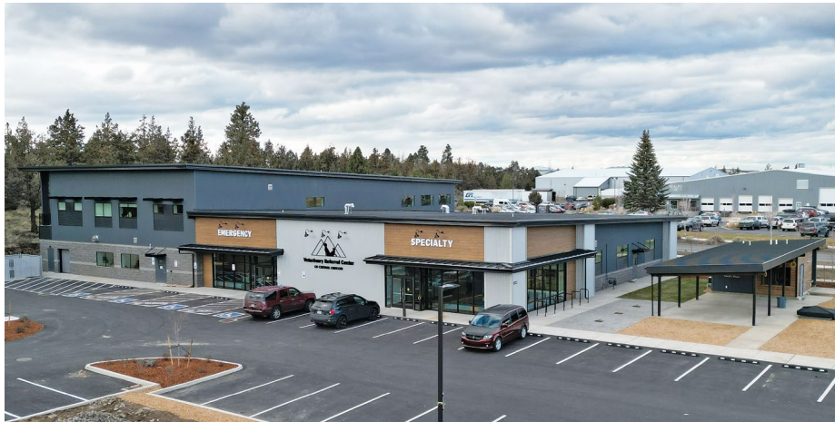
PHOTO | KEVIN SPENCER MASONRY
