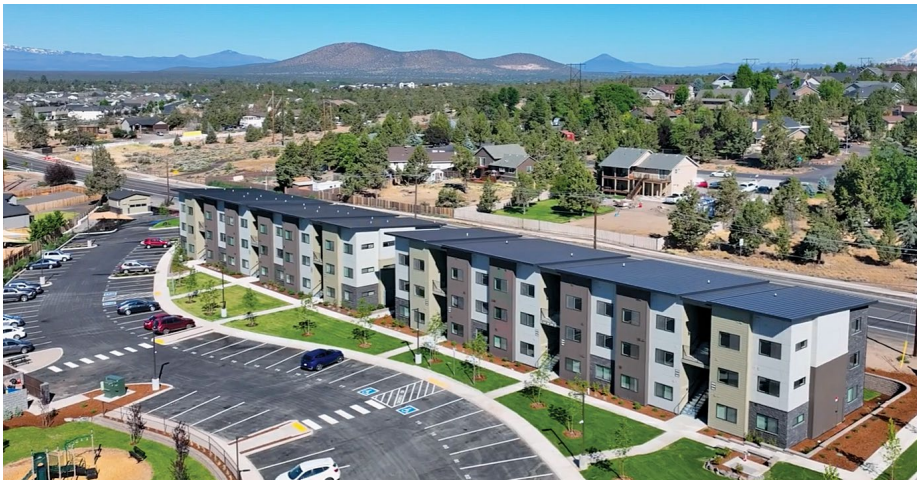
PHOTO | COURTESY OF STEELE ASSOCIATES ARCHITECTS
