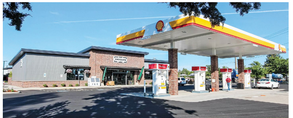
PHOTO | COURTESY OF STEELE ASSOCIATES ARCHITECTS
