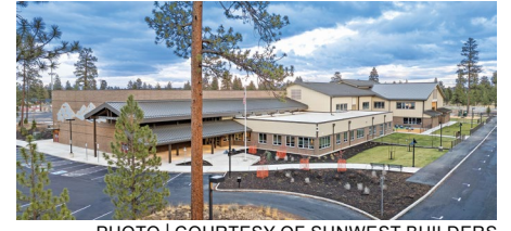
PHOTO | COURTESY OF SUNWEST BUILDERS
