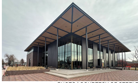
PHOTO | COURTESY OF STEELE ASSOCIATES ARCHITECTS
