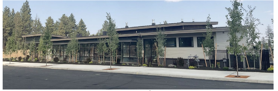
PHOTO | COURTESY OF STEELE ASSOCIATES ARCHITECTS
