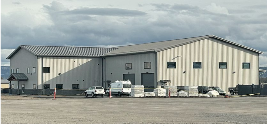
PHOTO | COURTESY OF KEVIN SPENCER MASONRY
