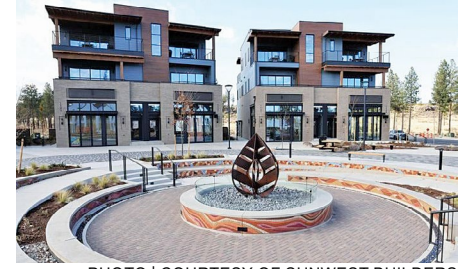
PHOTO | COURTESY OF SUNWEST BUILDERS
