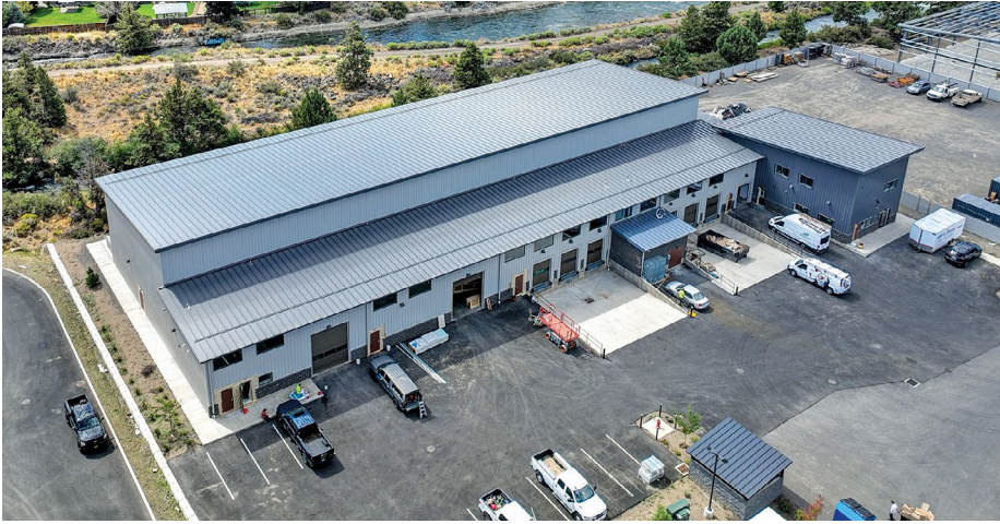
PHOTO | COURTESY OF KEVIN SPENCER MASONRY
