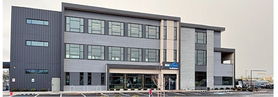
PHOTO | COURTESY OF SUNWEST BUILDERS
