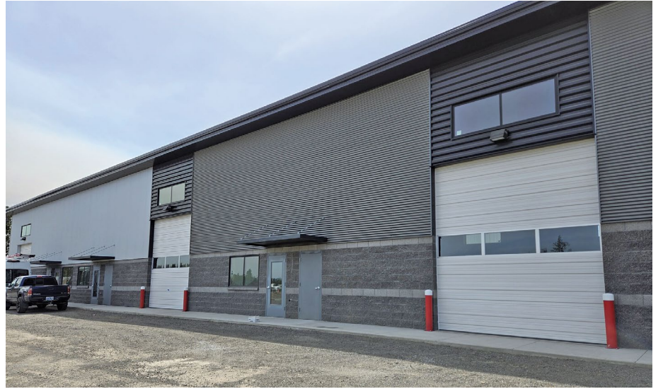
PHOTO | KEVIN SPENCER MASONRY
