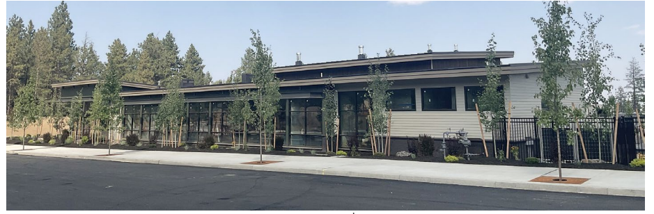
PHOTO | COURTESY OF STEELE ASSOCIATES ARCHITECTS
