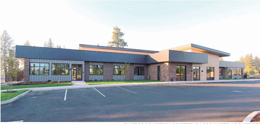
PHOTO | COURTESY OF STEELE ASSOCIATES ARCHITECTS
