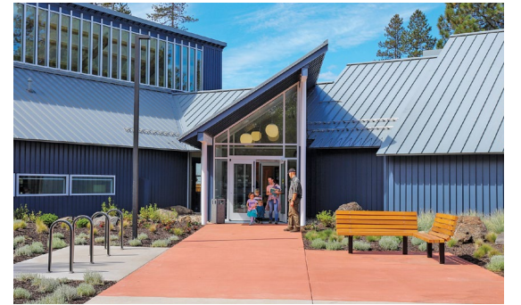
PHOTO | COURTESY OF SUNWEST BUILDERS
