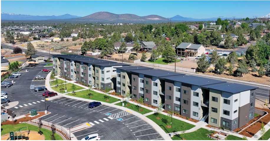
PHOTO | COURTESY OF STEELE ASSOCIATES ARCHITECTS
