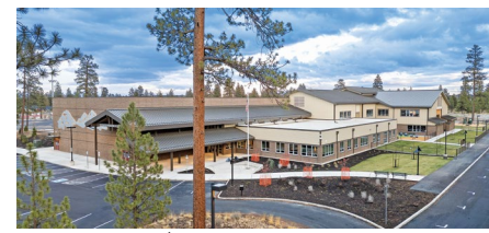
PHOTO | COURTESY OF SUNWEST BUILDERS
