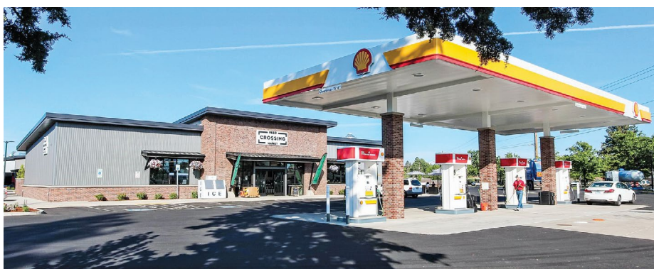
PHOTO | COURTESY OF STEELE ASSOCIATES ARCHITECTS
