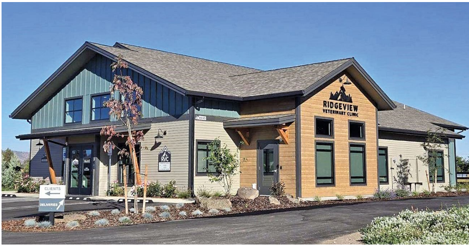
PHOTO | COURTESY OF STEELE ASSOCIATES ARCHITECTS
