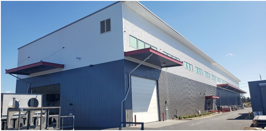
PHOTO | COURTESY OF SUNWEST BUILDERS
