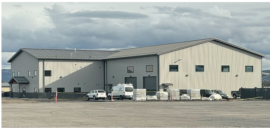
PHOTO | COURTESY OF KEVIN SPENCER MASONRY
