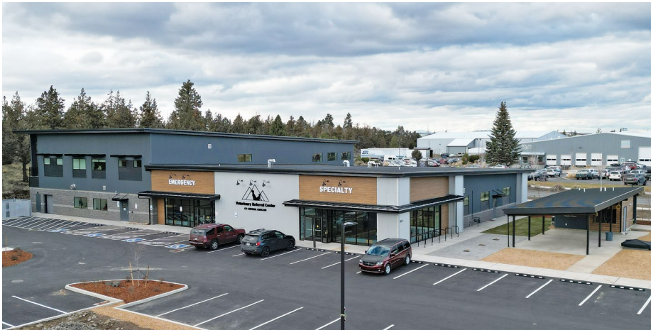
PHOTO | KEVIN SPENCER MASONRY
