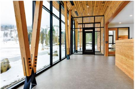
THE ROOF SYSTEM IN THE KAMIAH SUPERVISOR'S OFFICE IS COMPRISED OF MASS TIMBER CLT, EXTERIOR BEARING WALLS AND GLULAM BEAM/COLUMN SYSTEMS
