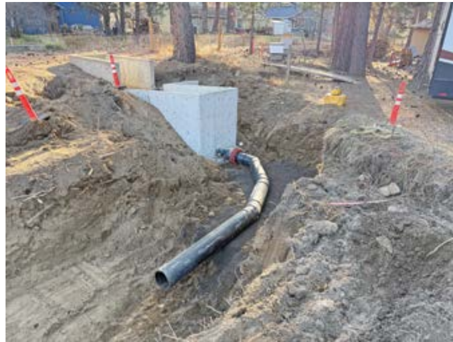
THE LUNDY DITCH PIPING PROJECT SOUTH OF BEND HAS MODERNIZED A NEARLY 100-YEAR-OLD PRIVATE IRRIGATION SYSTEM BY CONVERTING APPROXIMATELY 4,000 FEET OF OPEN, UNLINED DITCH INTO A CLOSED-CONDUIT PIPELINE. THE PROJECT NOT ONLY BENEFITS THE WATER RIGHT HOLDERS AND ADJACENT LANDOWNERS BUT ALSO SETS A PATHWAY FOR THE FURTHER ADVANCEMENT OF IRRIGATION MODERNIZATION IN THE AREA | PHOTOS COURTESY OF MORRISON-MAIERLE
