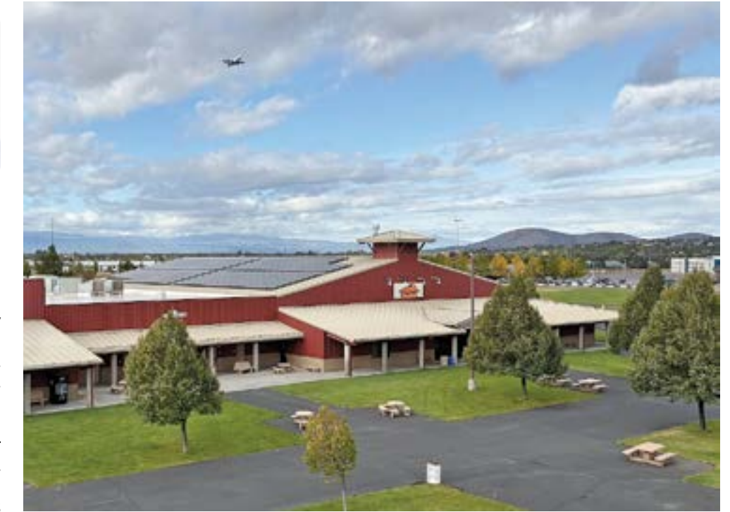
PHOTO | COURTESY OF E2 SOLAR
