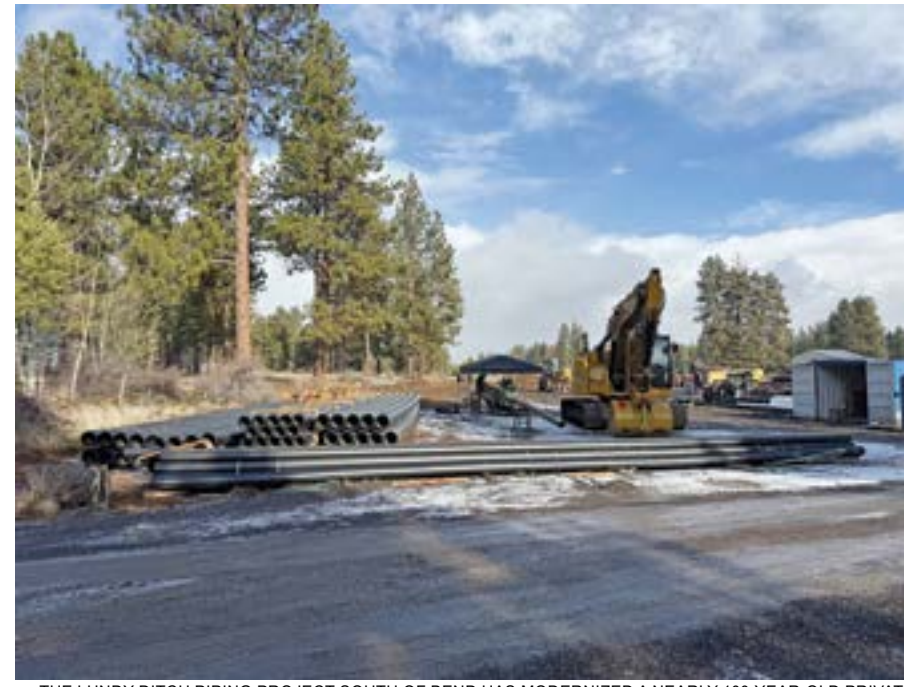
THE LUNDY DITCH PIPING PROJECT SOUTH OF BEND HAS MODERNIZED A NEARLY 100-YEAR-OLD PRIVATE IRRIGATION SYSTEM BY CONVERTING APPROXIMATELY 4,000 FEET OF OPEN, UNLINED DITCH INTO A CLOSED-CONDUIT PIPELINE. THE PROJECT NOT ONLY BENEFITS THE WATER RIGHT HOLDERS AND ADJACENT LANDOWNERS BUT ALSO SETS A PATHWAY FOR THE FURTHER ADVANCEMENT OF IRRIGATION MODERNIZATION IN THE AREA | PHOTOS COURTESY OF MORRISON-MAIERLE
