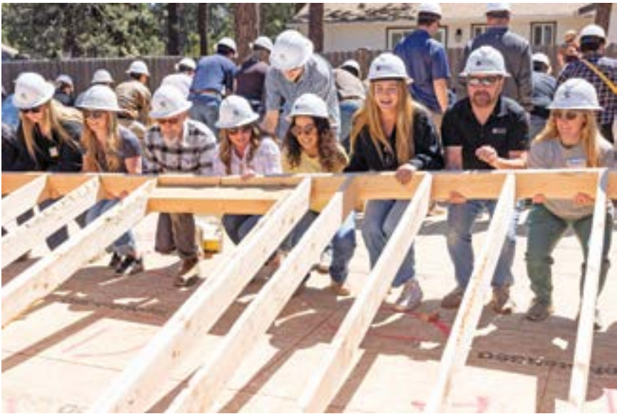
LOCAL NONPROFIT FIRST STORY, ALONGSIDE PARTNERS SUCH AS HAYDEN HOMES, NEIGHBORIMPACT, AND REGIONAL LEADERS, WORKED TOGETHER TO BUILD AND RAISE THE WALLS OF A NEW HOME FOR A BEND FAMILY IN MAY OF 2026 | PHOTO COURTESY OF FIRST STORY
